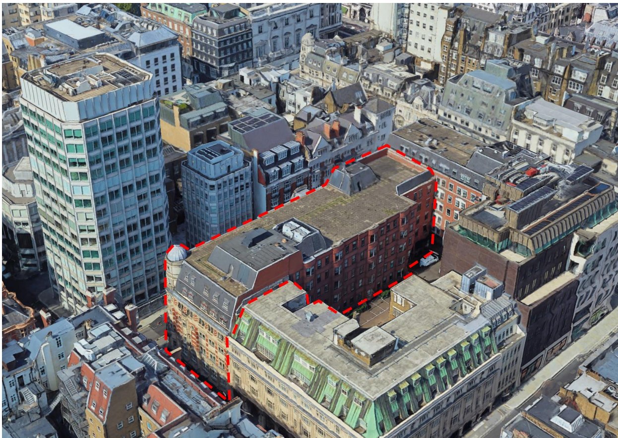
Ryder Court Aerial View
